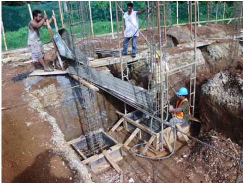
Construction side of the new NEOC.
