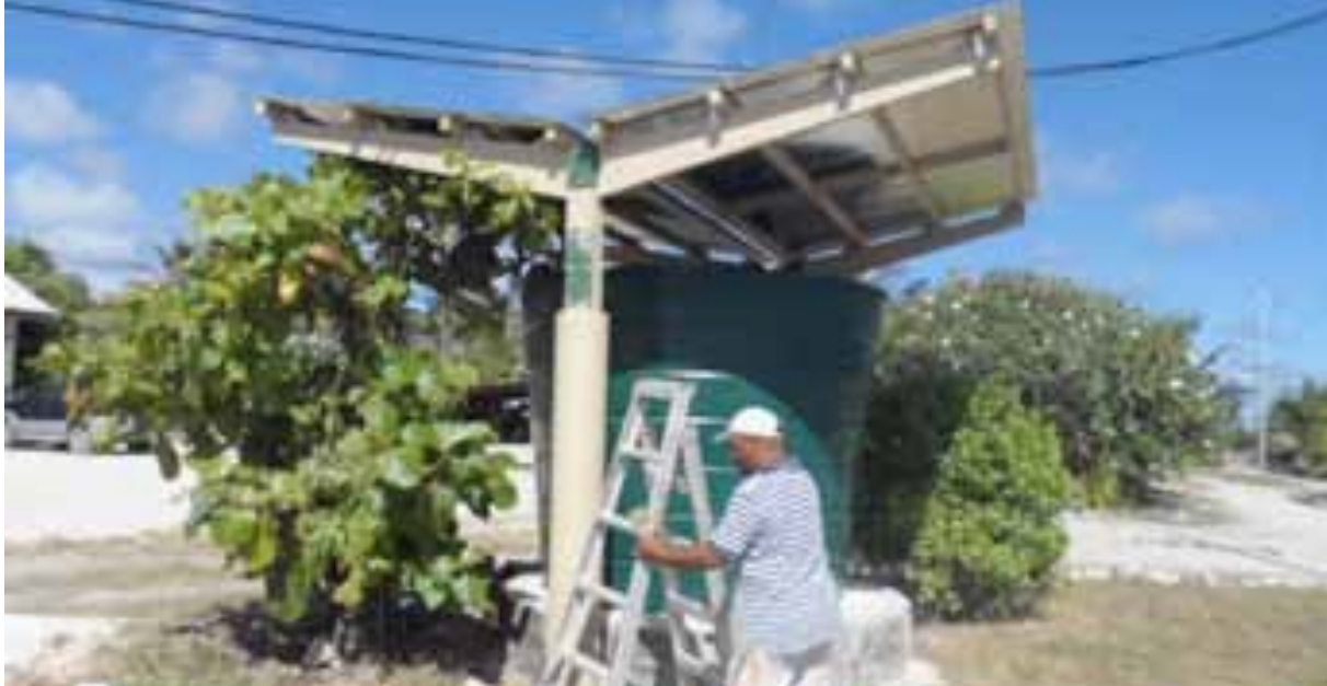
Rainwater catchment almost completed.
