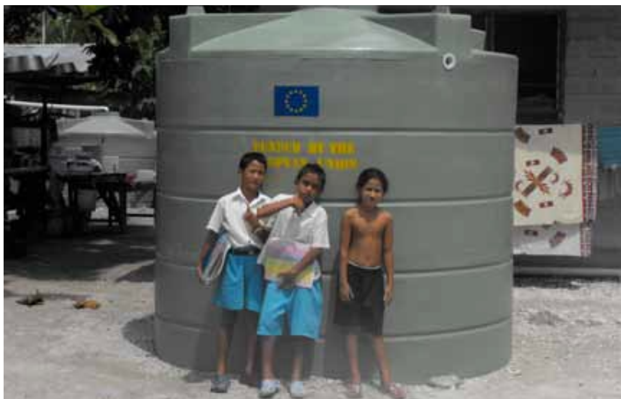
Newly installed water tank in Tuvalu funded by the B-Envelope Project.
