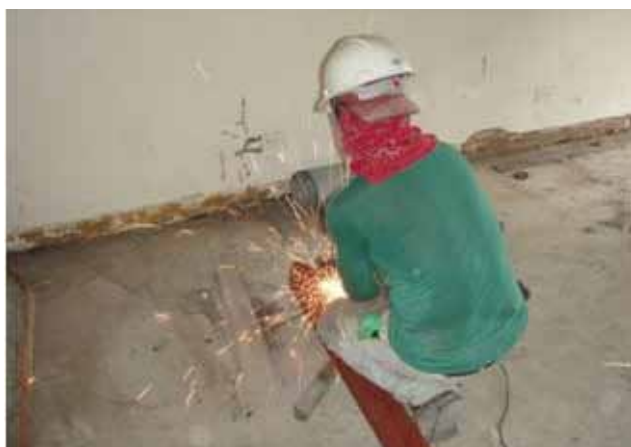
Channel cutting at the new EOC, Kosrae.
