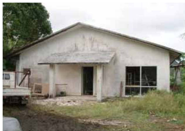
The new Kosrae State EOC under construction.
