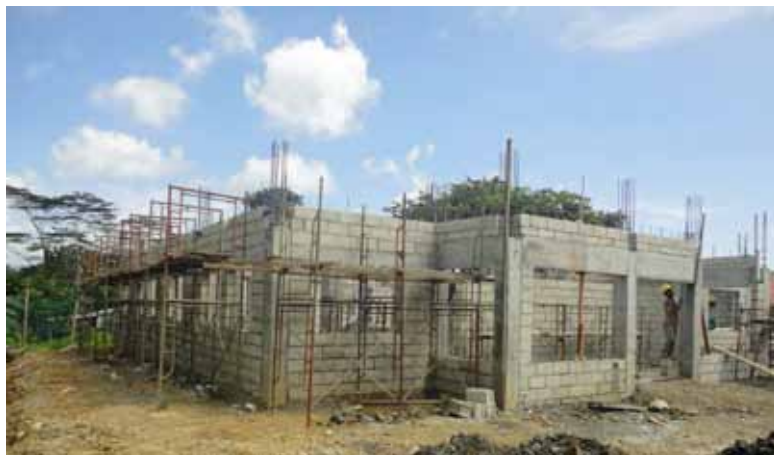
Construction of the National Emergency Operation Centre in Palikir, Pohnpei.
