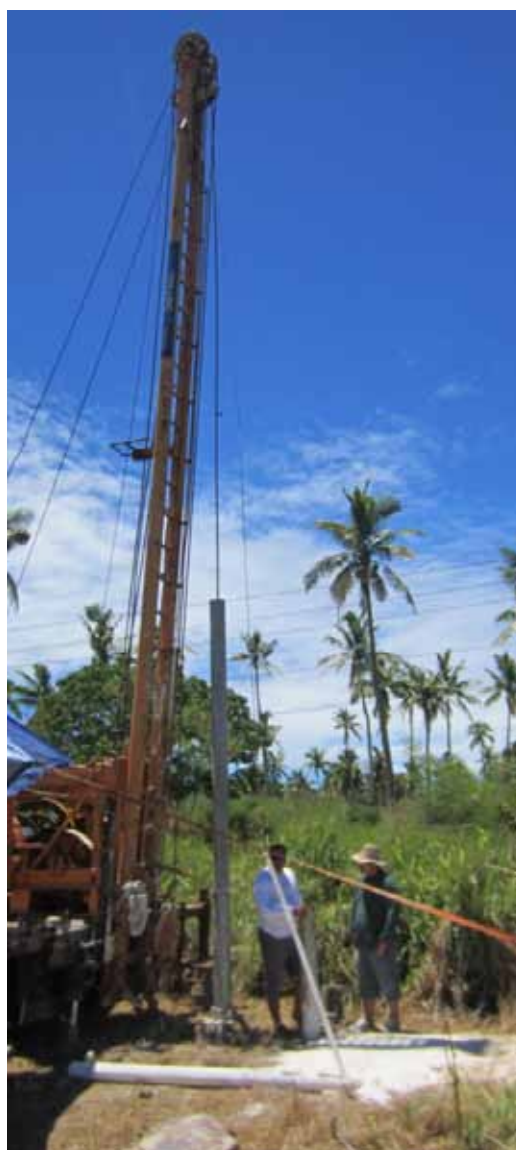
Borehole drilling at Fu'amotu.
