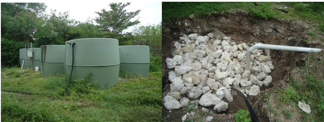
Figure 6. Sewage treatment Plant at Nauru Primary School with Effluent Dispersal Pit
