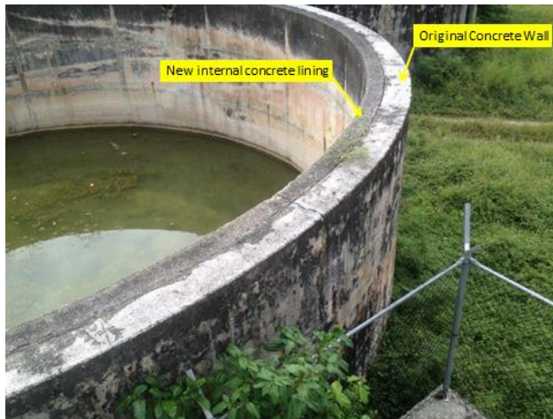
Figure 30. Past Remedial Works at Command Ridge Tanks
