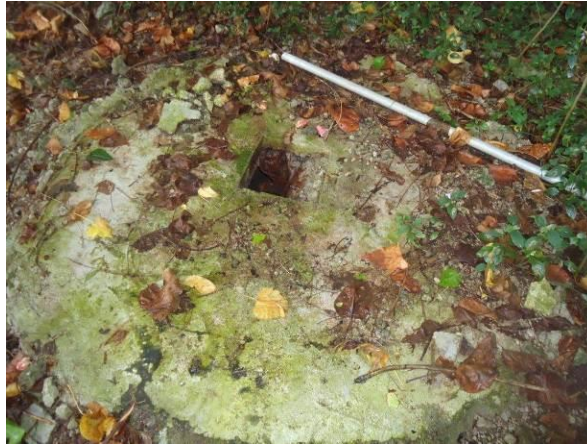
Figure 7. Cesspit at Nauru Primary School Receiving the School's Sewage
