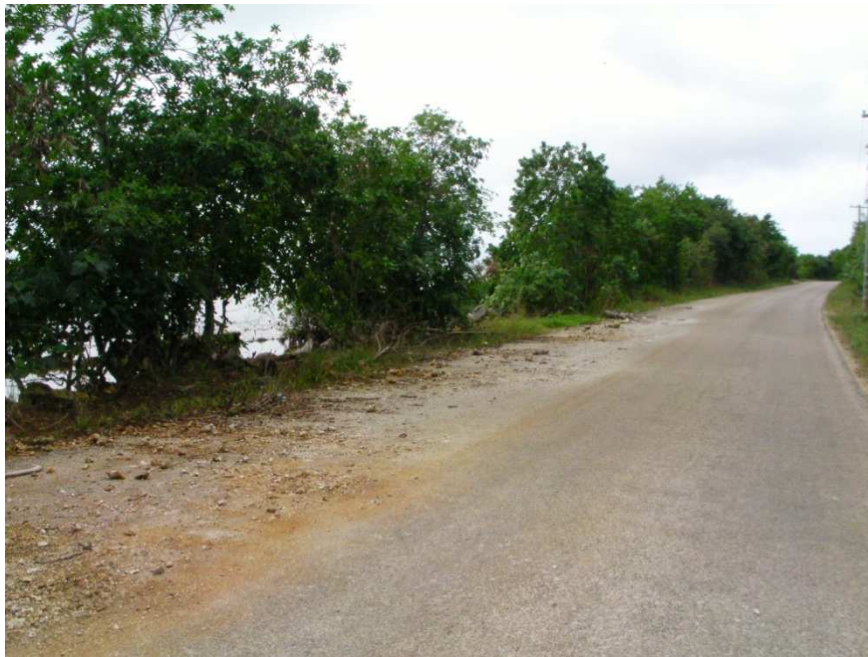
Figure 2.8. Over-topping along the eastern part of the 390 m long trial site.
