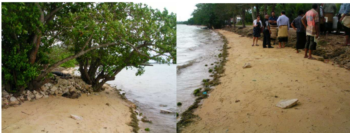
Figure 2.2. A fillet of sand on the northern side of a small groyne in Makaunga Village.
