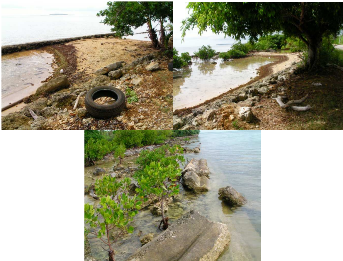
Figure 2.6. Tombolos and mangroves growing in the lee of failed sections of the seawall.
