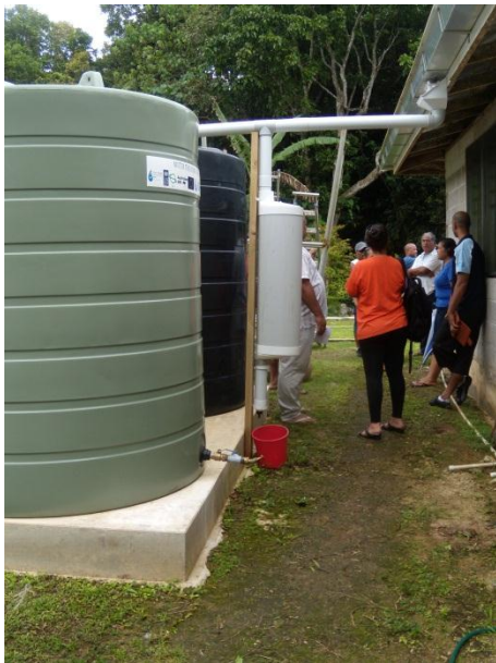
Installed water tank with first flush device
