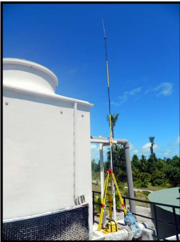
Figure 8. To increase radio coverage, the radio antenna was mounted on top of the Public Utilities water tower.
