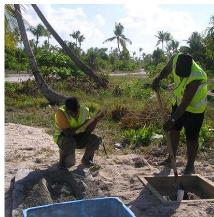
Figure 16. Community members assisting with the construction of piezometers on the Bonriki water reserve
