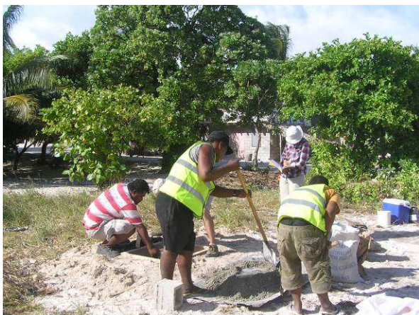
Figure 16. Community members assisting with the construction of piezometers on the Bonriki water reserve
