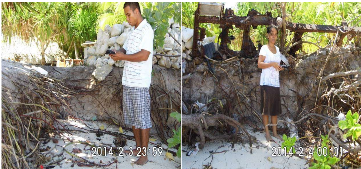
Figure 4: At the ocean side of Abeton's house.
