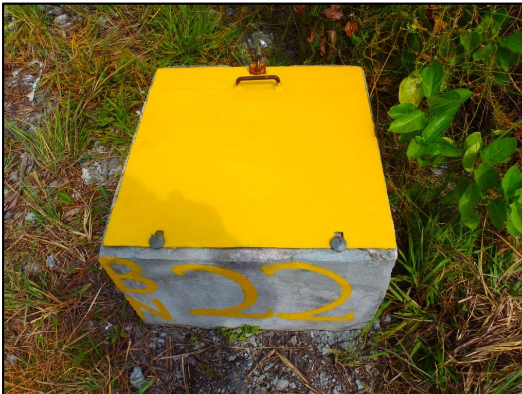
Figure 14: The steel monitoring borehole lids have been repainted to extend its life.
