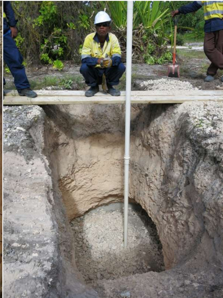
Figure A5.28: Gravel pack and piezometer placement.
