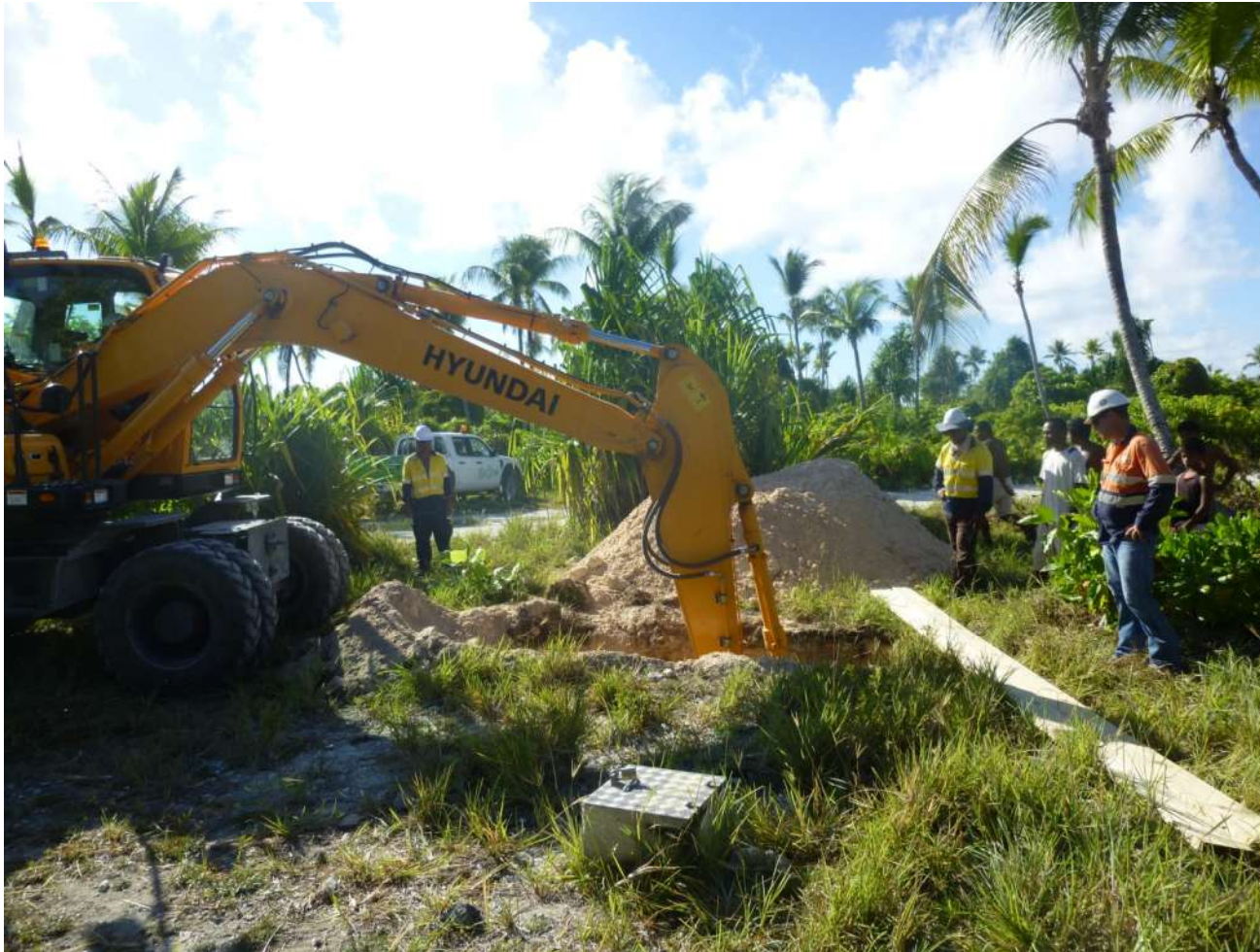
Figure A5.24: Excavator digging piezometer pit – BN1.
