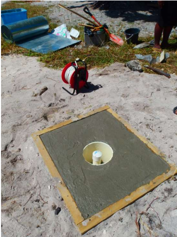
Figure A5.30: Construction of monitoring headworks – BN15.
