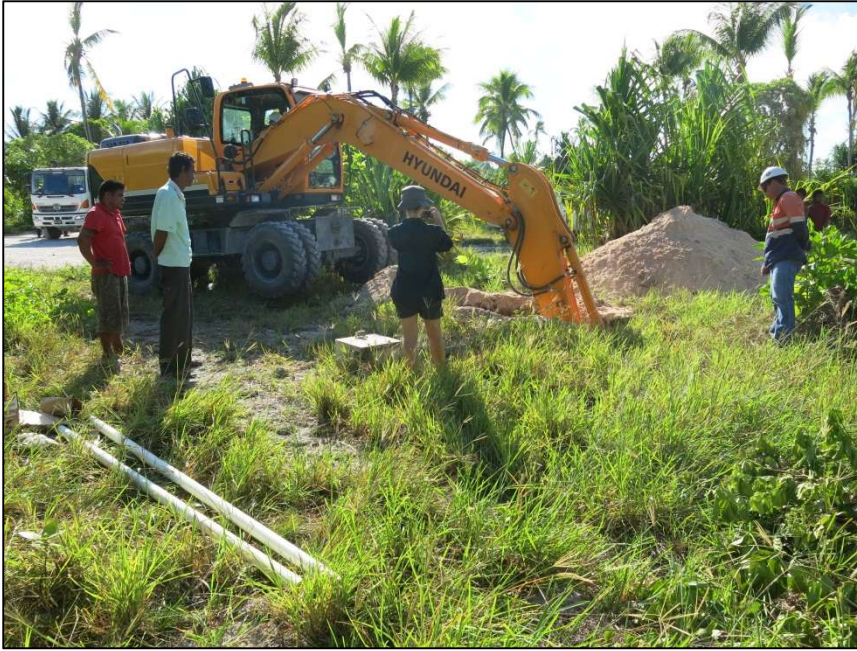
Figure A5.2: Digging at piezometer – BN1B, Bonriki (14/11/13).
