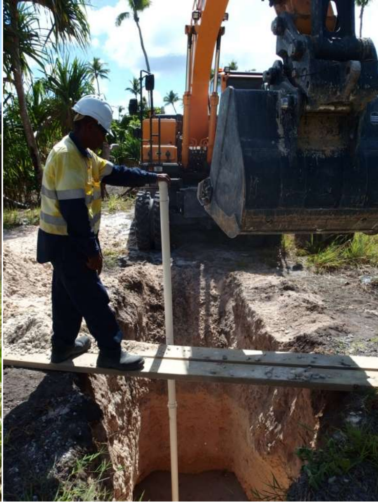
Figure A5.26: Positioning of piezometer – BN23.
