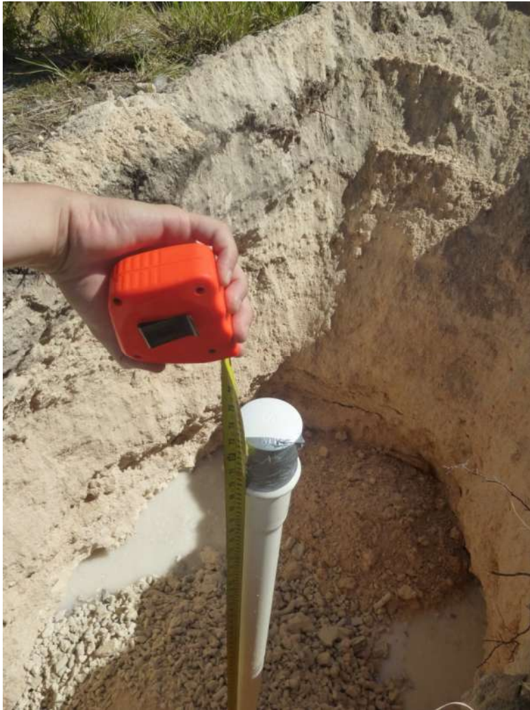
Figure A5.27: Measurement of gravel pack.
