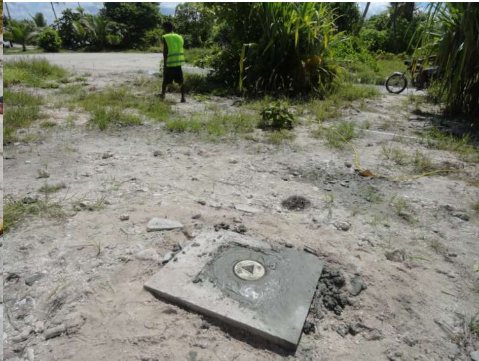
Figure A5.31: Finished borehole cover – BN1.
